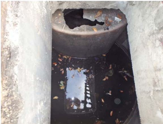
Deteriorated Baffle and Broken Apron in Phase I
