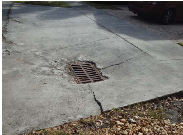
Deteriorated Baffle and Broken Apron in Phase I
